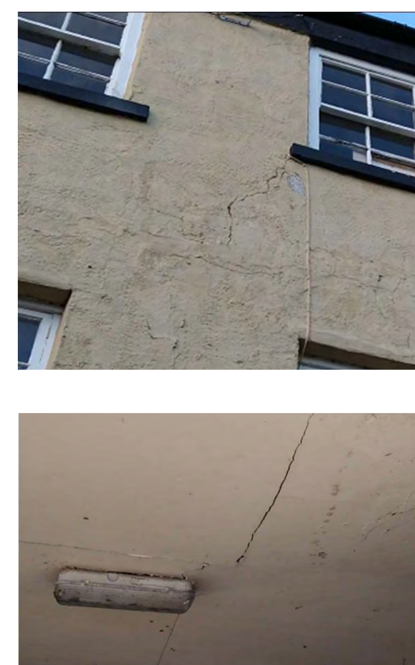
Postchaise, the front elevation has moved away from the rest of the building. There is cracking at the interface between the front wall and the internal walls at both first and second floor.
