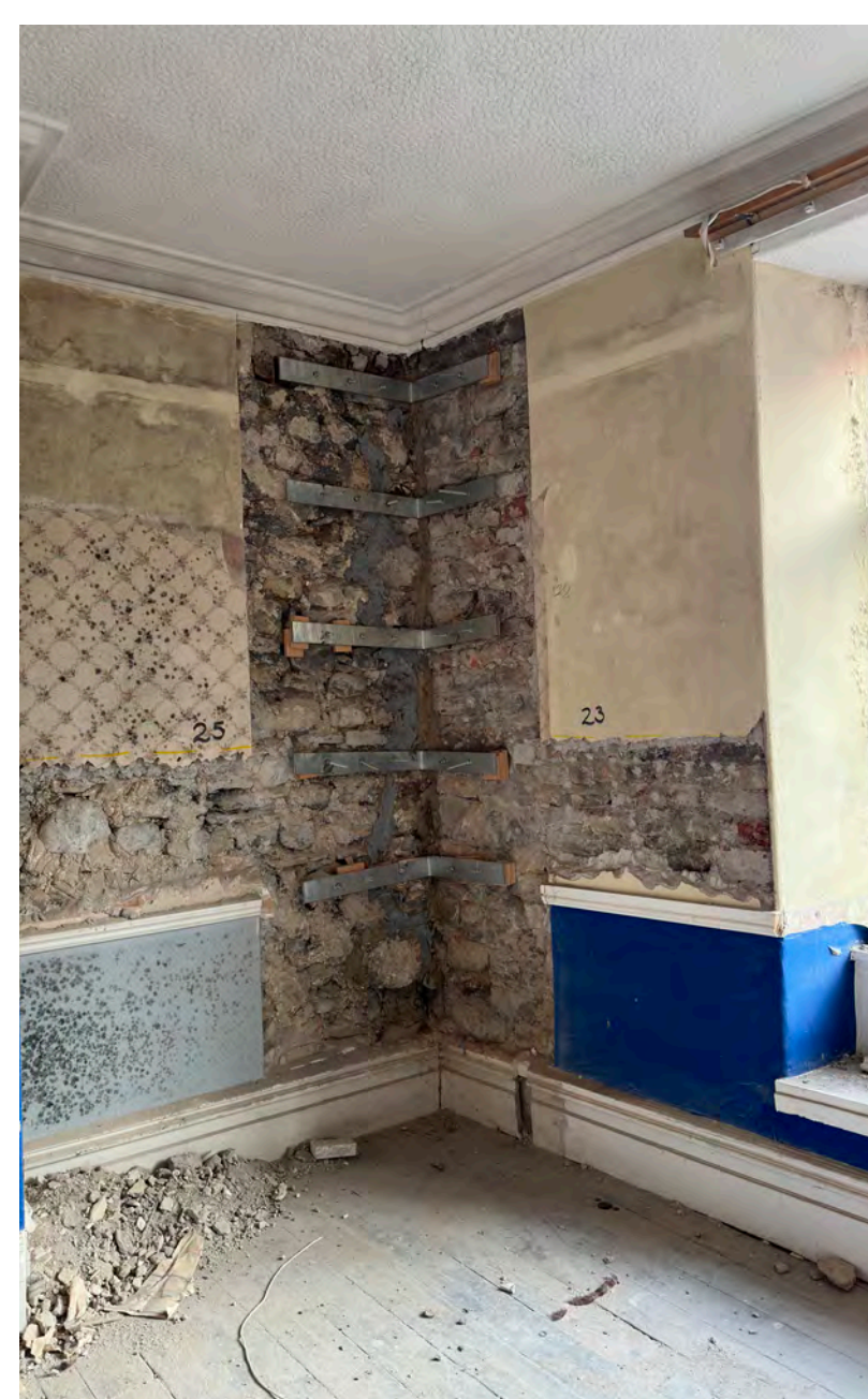
Queens Head movement of the front elevation and crack in the facade, internal strapping support. Internal condition above, damage ranges from repairs to structural demolition.
